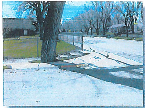
Handicap ramp added where only steps initially existed
